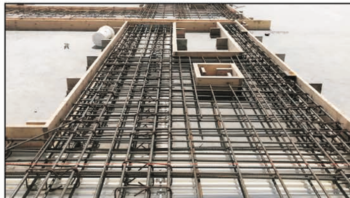
Being molded: concrete tilt-up walls with steel reinforcement throughout.
