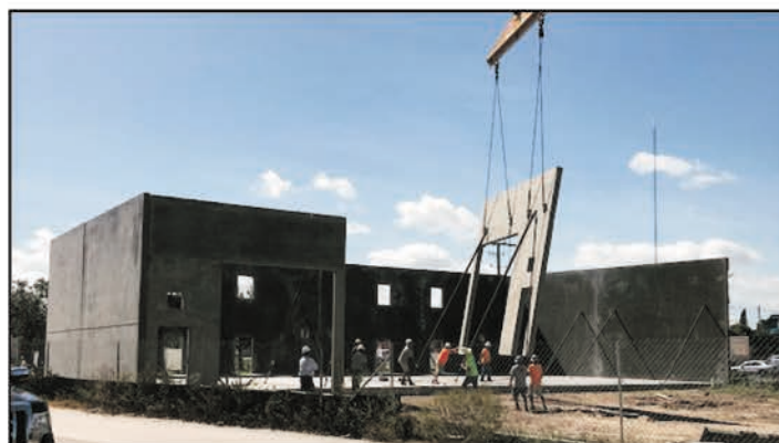
A solid concrete tilt-up wall is placed in position.
